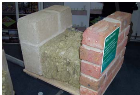
Figure 2d: Section through a very highly insulated external wall with a heavyweight concrete inner leaf for good thermal mass. This provides excellent year-round thermal performance by creating an optimised combination of energy flow and storage. (Photo taken during study tour at BedZED, UK)
